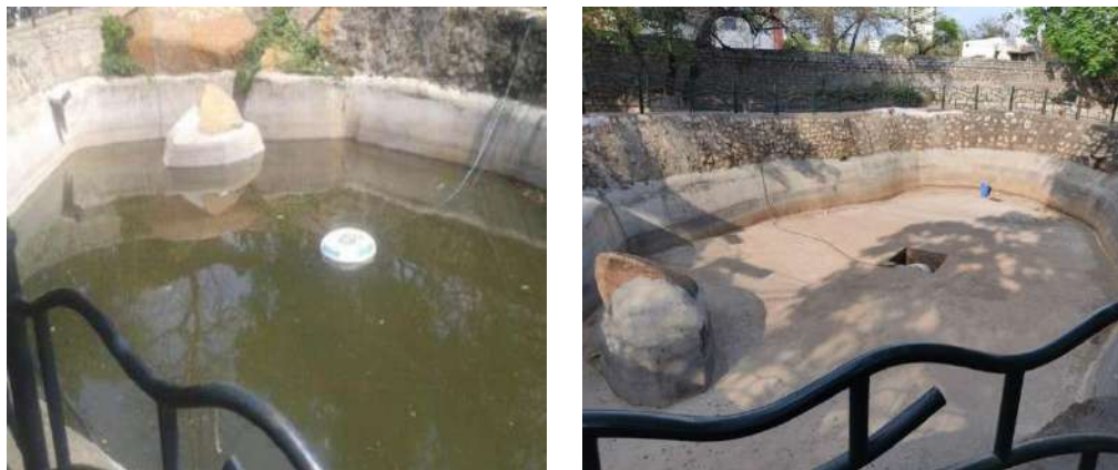
Figure 4-7: Rain water harvesting pond
