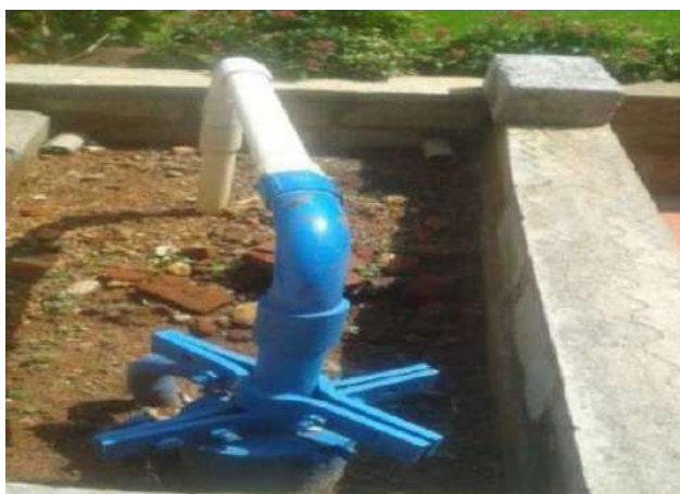
Figure 4-12: Point recharge for a Bore well
