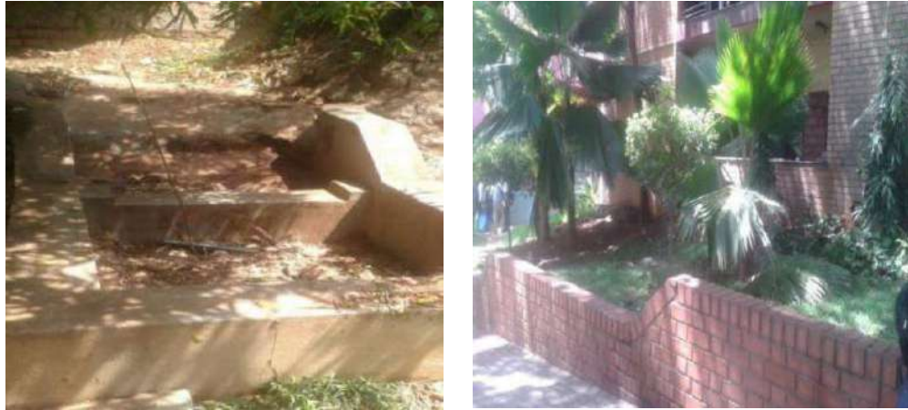
Figure 4-6: Trenches and bunds in the campus
