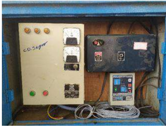
Figure 4-3: Level controller switch
